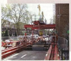
opening with special bridging mats for additional ground support. The strand jack frame was preassembled ready for operation and to reduce rigging time. Stuart Rawcliffe, JB Rawcliffe & Sons, said. "The redundant transformer was lifted from its operating position 8 m below ground level and loaded directly to transport in one simple and safe operation," a JB Rawcliffe spokesperson said. The replacement transformer was then lifted into position using the same method.
